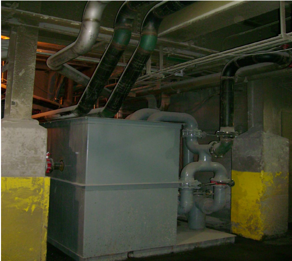
Figure 8. The recirculation tank, piping, and strainers.
