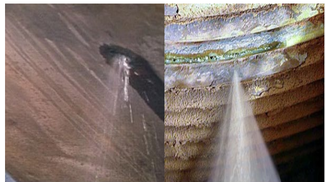
Figure 15. The above pictures show a typical leak in a spray-cooling roof (left) compared to a pressurized tubular system (right), 5 GPH vs. 16,000 GPH.
